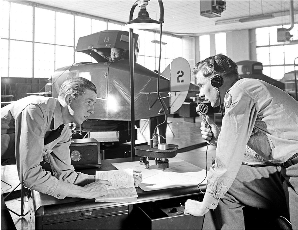
Patented in 1929, the **Link trainer** permitted pilots to practice more deeply, to stop, struggle, make errors, and learn from them. During a few hours in a Link trainer, a pilot could “take off” and “land” a dozen times on instruments. He could dive, stall, and recover, spending hours inhabiting the sweet spot at the edge of his capabilities in ways he could never risk in an actual plane.
