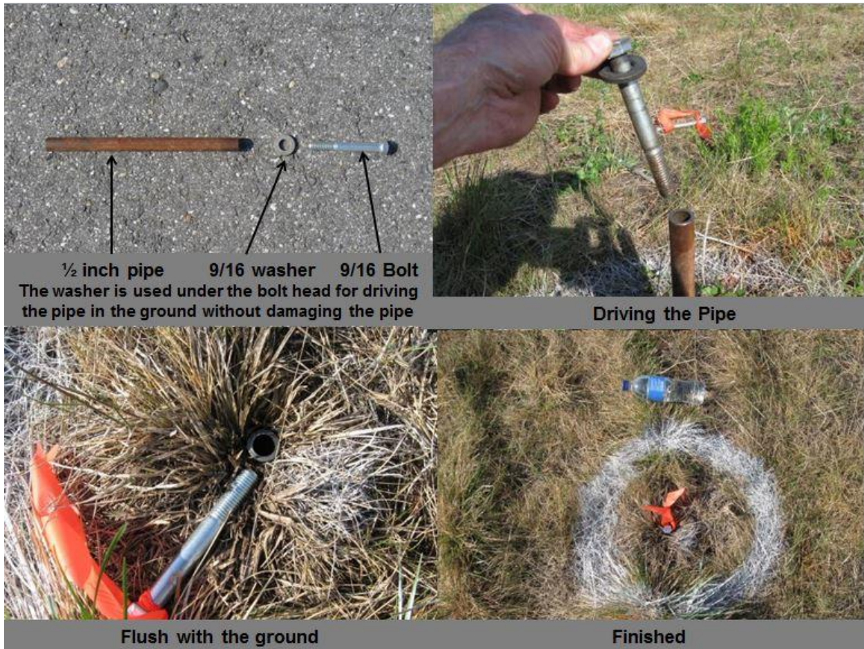
Figure B-5. Driving pipes off the edge of the runway to permanently establish reference points greatly speeds up the marking process during painting projects. The bolt stays in the pipe, and is marked with flagging to make it easier to find.
