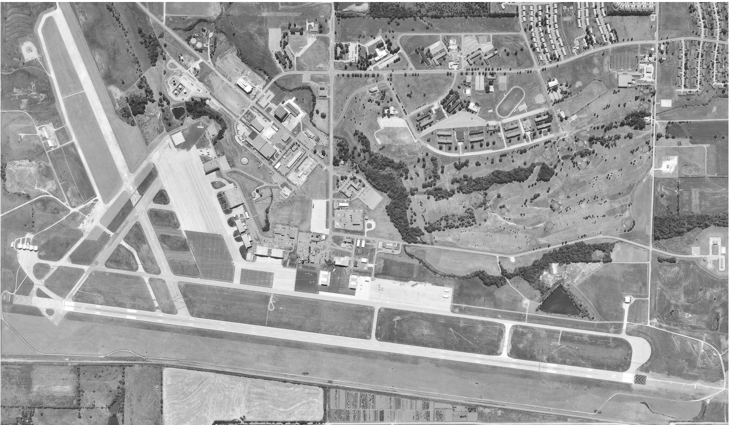
Figure 4: Aerial View of Richards-Gebaur Memorial Airport, Kansas City, Missouri
