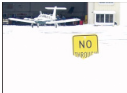
Snow obscured taxiway information sign.
