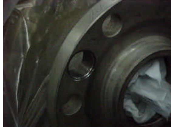
FIGURE 12 CORE SAMPLE HOLE AFTER CHAMFERING
